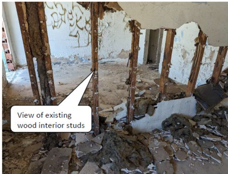
Photo No. 6 – View of interior studs.
