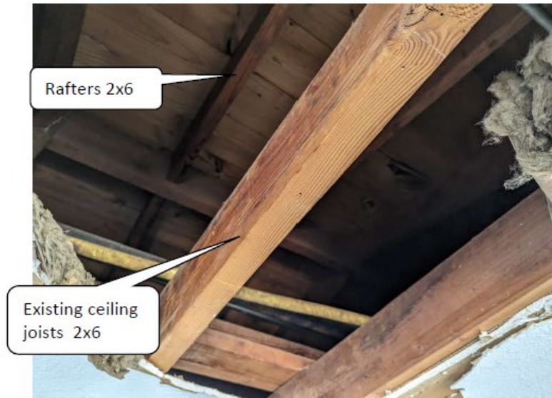
Photo No. 8 – View of roof framing.
