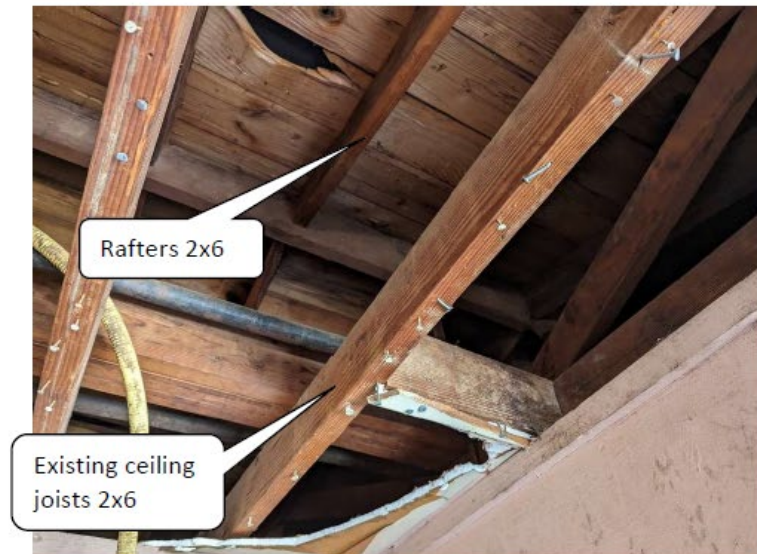
Photo No. 9 – View of roof framing.
