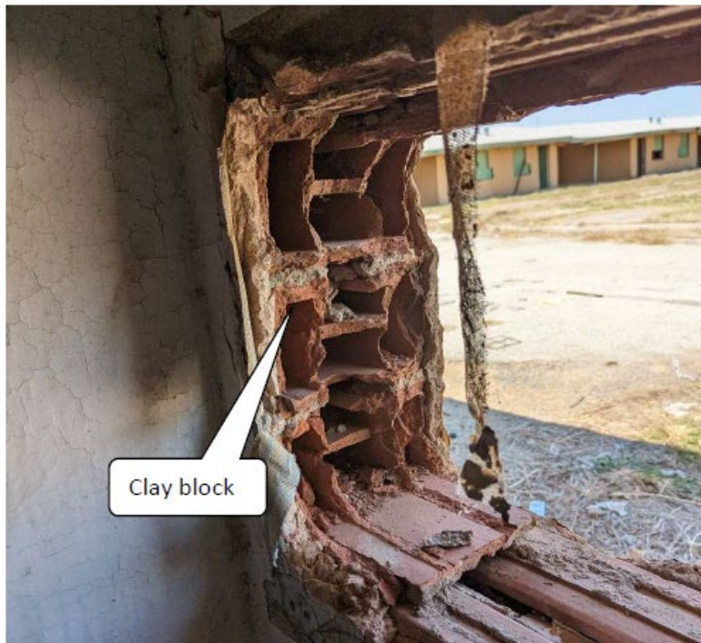
Photo No. 10 – View of the exterior wall construction.
