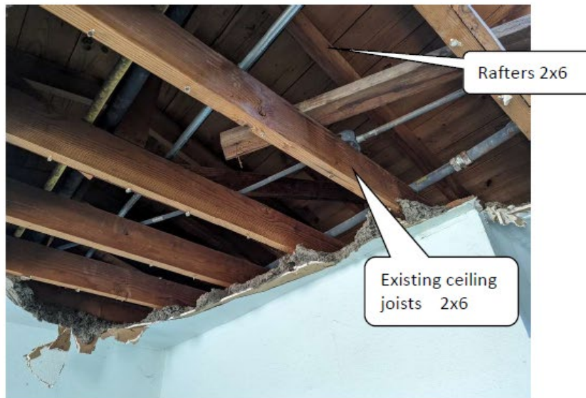
Photo No. 7 – View of the roof framing.
