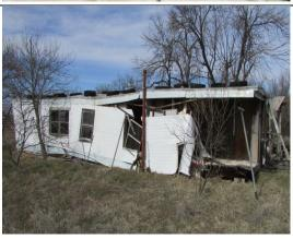
**Exterior Walls:** Cracks / holes in walls, large hole on the West side of the structure, missing members, deteriorated members, loose members, listing walls, several areas of exposure to outside elements.
