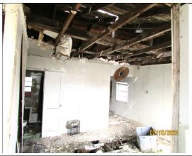
**Exterior Walls:** Cracks / holes in walls, missing members, deteriorated members, loose members, listing walls, several areas of exposure to outside elements.
