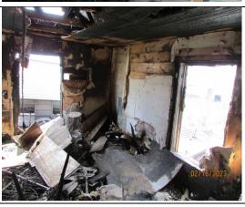
Exterior Walls: Significant fire damage throughout, cracks / holes in walls, missing members, deteriorated members, loose members, listing walls, several areas of exposure to outside elements. Roof: Significant fire damage, deteriorated / water damaged members, roof has caved in, multiple holes. Interior Walls / Ceiling: Significant fire damage throughout, broken sheetrock / holes in wall and ceiling, deterioration / water damage throughout, areas of exposure to outside elements.
