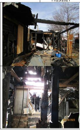
**Exterior Walls:** Fire / smoke damage, cracks / holes in walls, missing members, deteriorated members, loose members, listing walls, several areas of exposure to outside elements.
