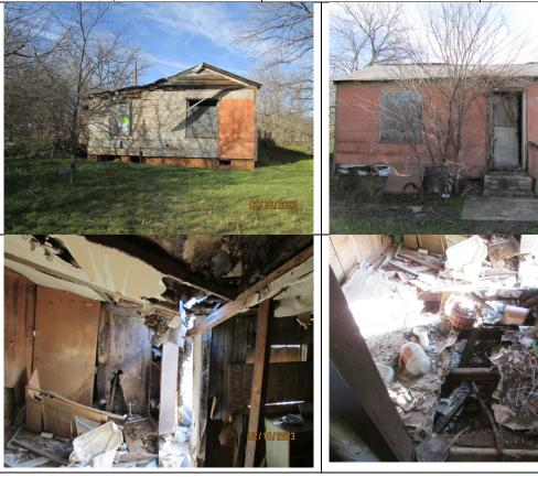
**Exterior Walls:** Crack / holes in walls, deteriorated structural members, loose members, protective coating/paint missing.
