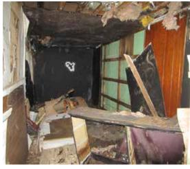
**Exterior Walls:** Cracks / holes, loose members, missing siding. **Interior Walls/Ceiling:** Water damage, broken sheetrock / holes in wall & ceiling, interior vandalized.
