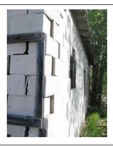
**Exterior Walls:** Loose members, deteriorated structural members, cracks / holes in wall. **Interior Walls / Ceiling:** Holes in wall and ceiling, water damage.
