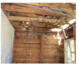
**Interior Walls / Ceiling:** Broken sheetrock / holes in wall and ceiling, ceiling collapsing, interior vandalized, water damage.
